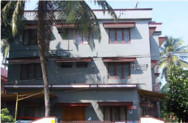
Ground floor of Future point, at Edipazhanji, Thiruvananthapuram
